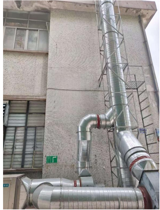
废气排放口DA001 (远照)
